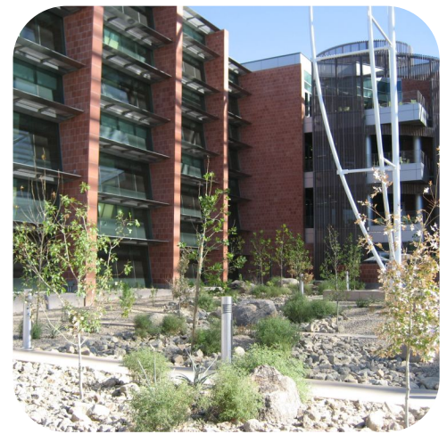
Medical Research Building
