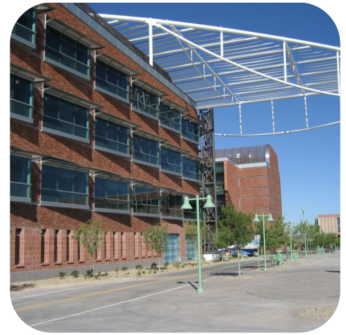
Thomas W. Keating Bioresearch Building
