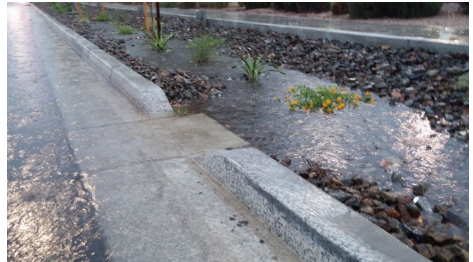
Curb Opening During Storm Event
