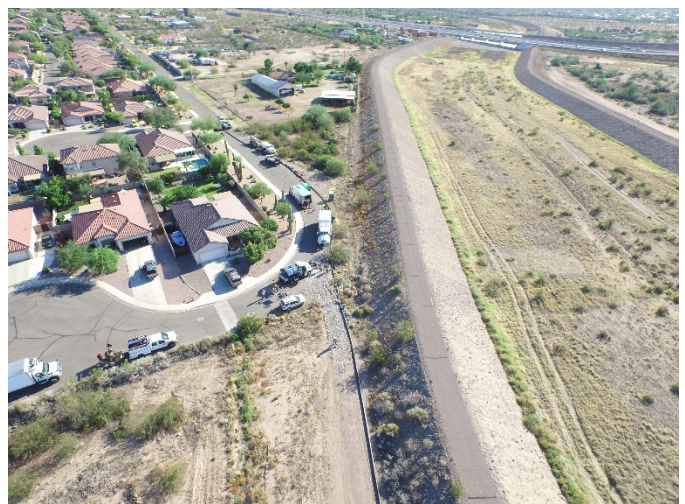
Aerial View of the Skunk Creek Levee System
