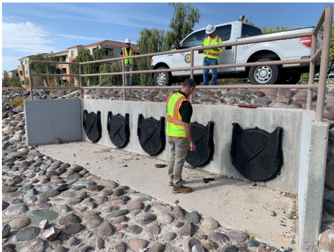
Five, 30-inch RCP Outlets
