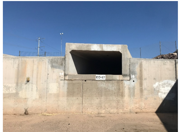
Concrete Box Culvert Outlet
