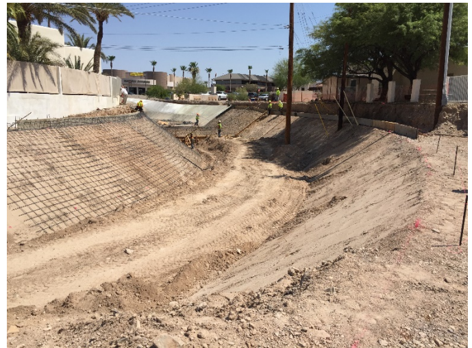
Broadwater Drain 1 – During Construction
