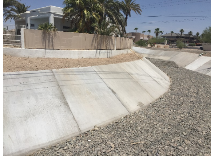
Broadwater Drain 1 – Post Construction
