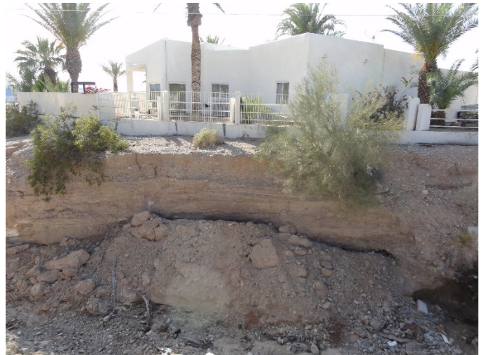
Broadwater Drain 1 – Pre-Construction
