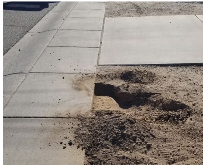
Locating of a Buried Manhole
