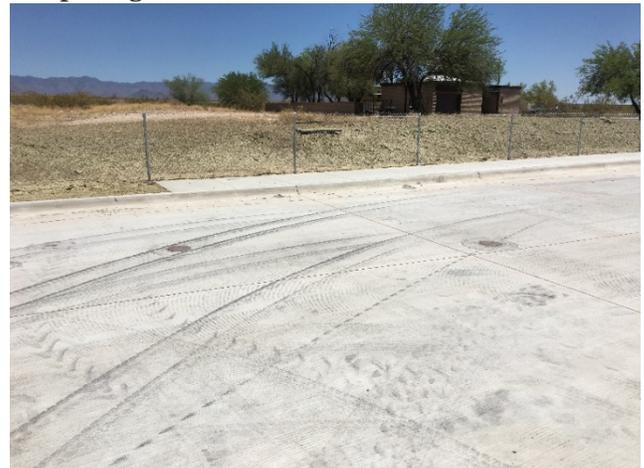
Septic system – caretaker's residence in background, septic tanks in middle, and tack welded cast iron lids in foreground
