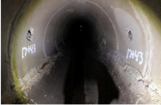
Storm drain with reference stations and inlet pipes
