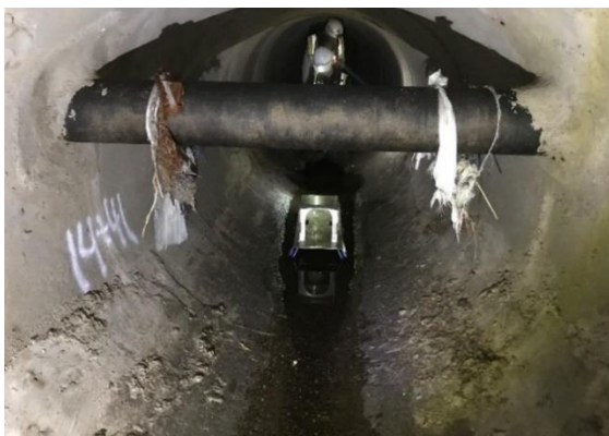
Sewer lateral spanning storm drain
