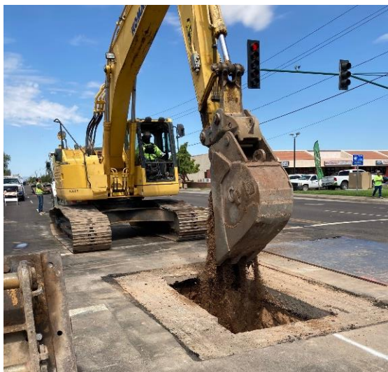
35th Avenue excavation
