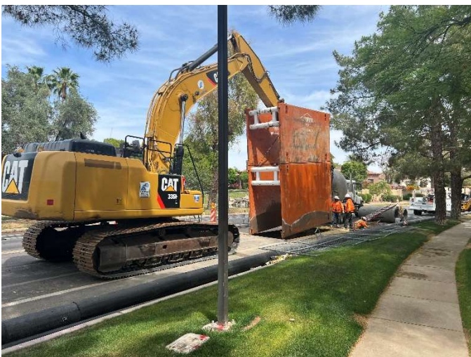
Construction along Jacaranda Parkway
