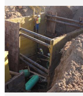
**Installing Large Sewer Structures:** Preparing to install a deep cast-in-place sewer junction structure (above), compared to a precast polymer concrete diversion structure (below).
