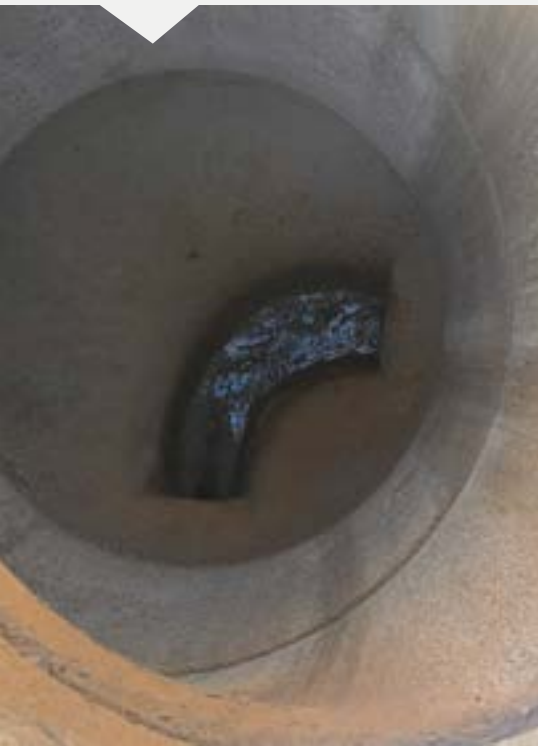
Bend in a manhole
