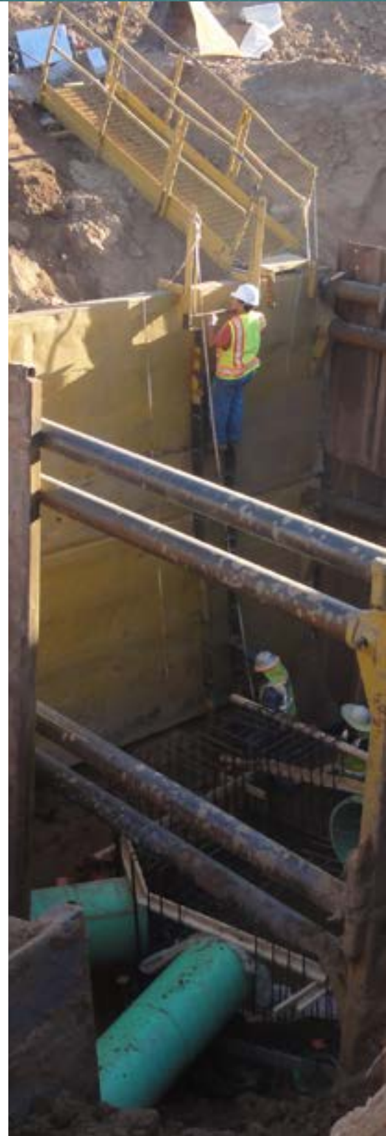
Installing a deep cast-in-place sewer structure
