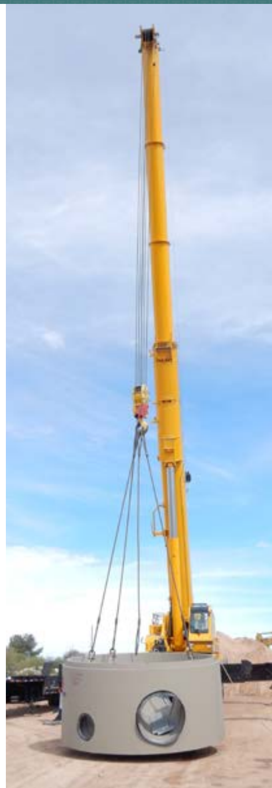
Preparing to place a large precast diversion structure
