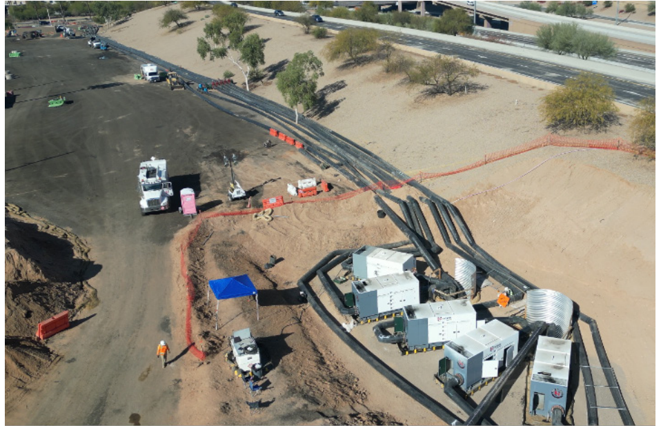
Figure 9 - Complex Bypass Pumping System Staged Near ADOT Loop 202
