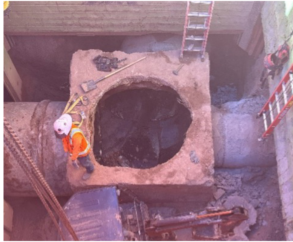
Figure 4 - Deteriorated Manhole
