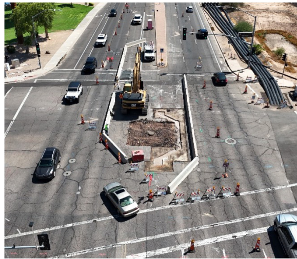
Figure 4 - Manhole Excavation
