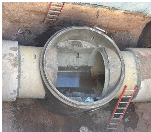
Figure 6 - New Polymer Manhole
