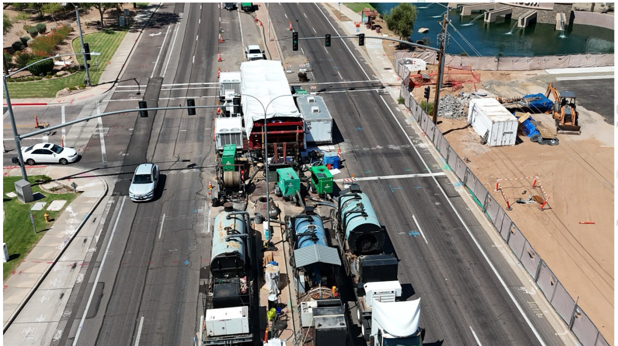
Figure 14 - Overview of CIPP Lining Installation
