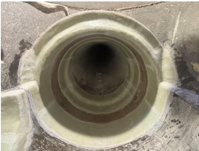
Figure 8 - Installed FRP Termination Seal
