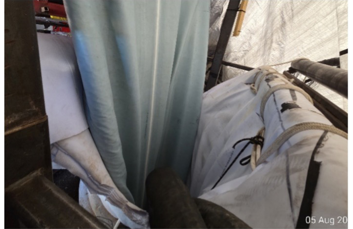
Figure 13 - Installing the CIPP Liner
