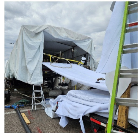
Figure 3 - CIPP Liner
