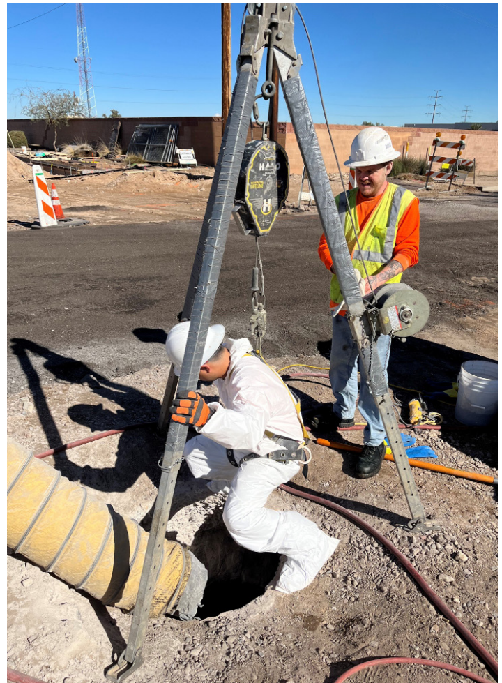
Manhole entry during a sewer assessment
